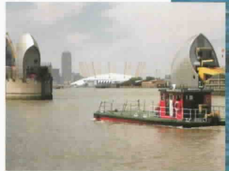
75 HP Hydromaster in continuous use on The Environment Agency - Barrier 1 work barge for over 17 years
